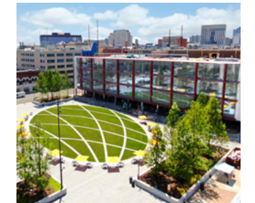
Bulletin Building Construction
