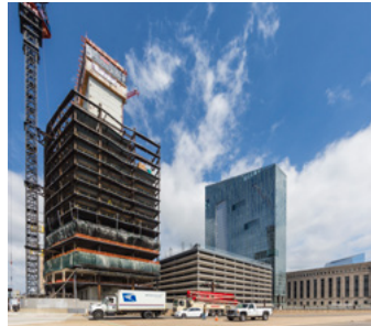
Construction of FMC Tower at Cira Centre South
